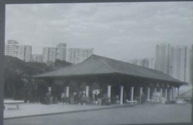
1966至2006年期間，舊卜公碼頭的鐵鑄桁架曾用作九龍摩士公園涼亭的上蓋。 The roof of the old Blake Pier served as the roof of a pavilion in the Morse Park in Kowloon from 1966 to 2006.
